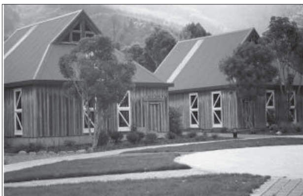
Anakiwa Outward Bound Bunkhouses
